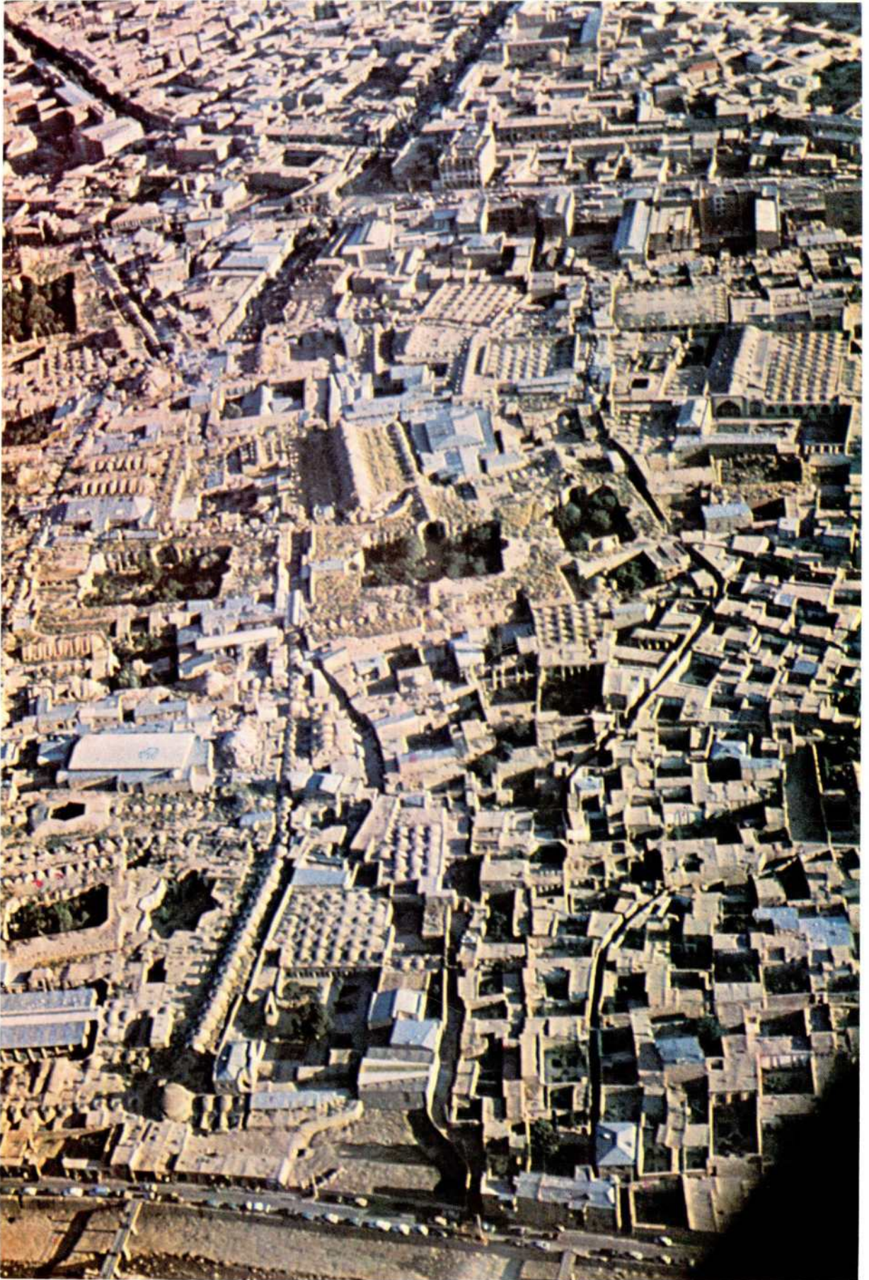
Tabriz: General view of the City
