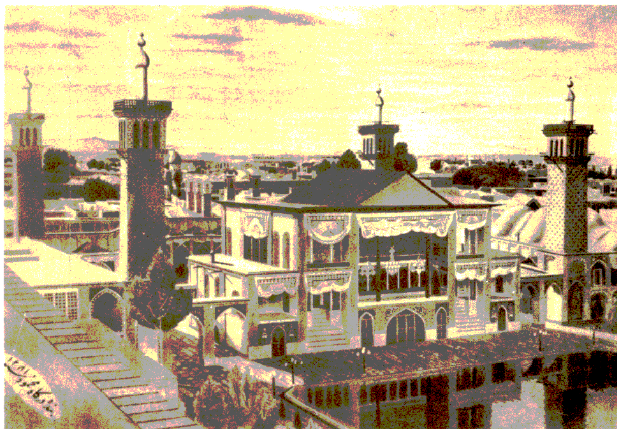
Teheran: Ventilation Building
