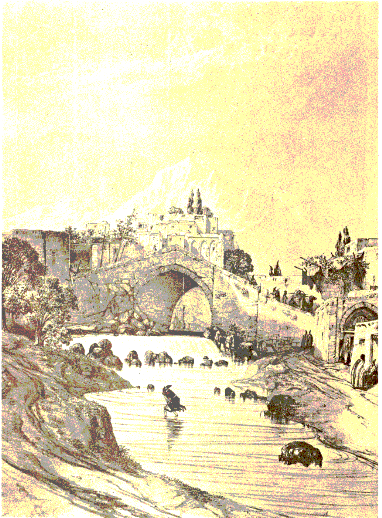
Hamadan: General View
